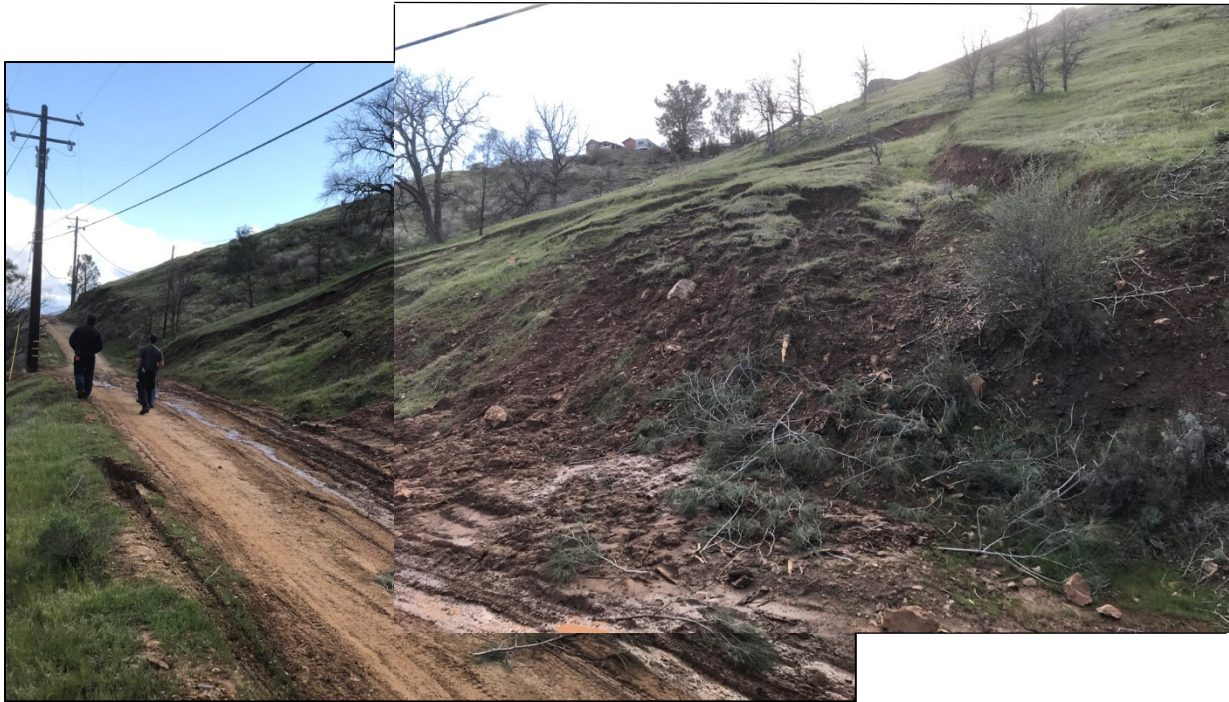
Photo I: Landslide (earth slide/flow) sourced from soil and colluvium exposed in old cut slope along Sierra Vista Drive.
